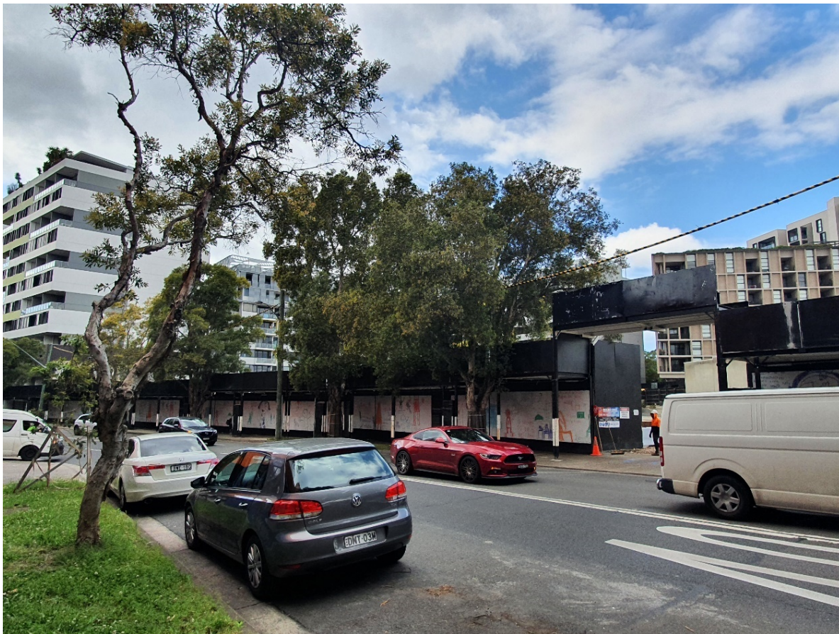
O'Dea Avenue frontage - looking east
