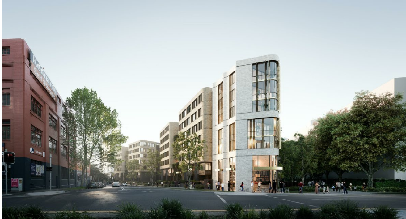
View along O’Dea Avenue – Building A in foreground
